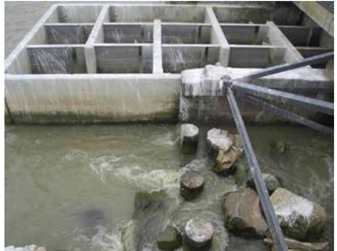
Rock-ramp and vertical slot fishways, Tauwichee Barrage
