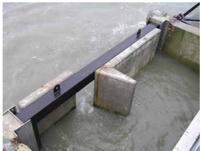
Entrance/exit to vertical slot fishway, Tauwichee Barrage
