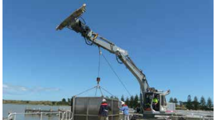
Placement of monitoring cage in existing fishway at Goolwa Barrage
