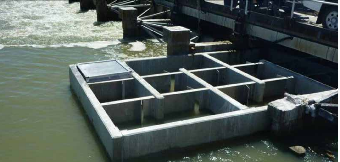
Existing vertical slot fishway at the Tauwichee Barrage
